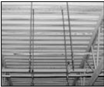
Figure 13: Suspension points with turnbuckles installed
